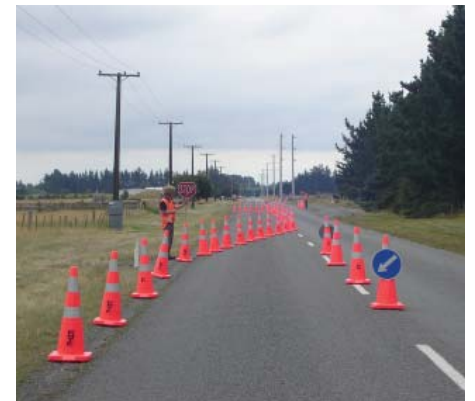
Example of side friction on approach to cone threshold at MTC Position
